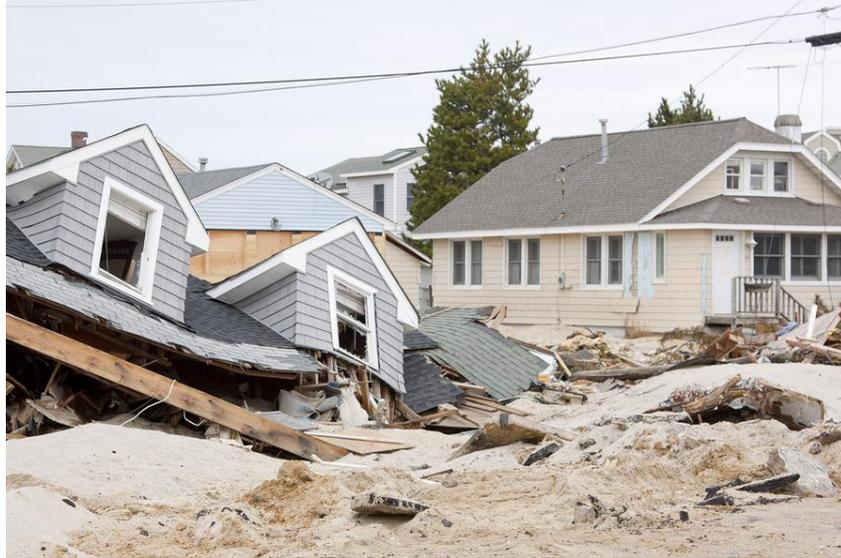
Figure 1: Storm Surge Damage During Superstorm Sandy
